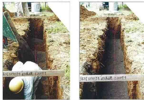
(敷砂状況) (敷砂完了)
