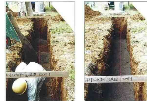
(敷砂状況) (敷砂完了)
